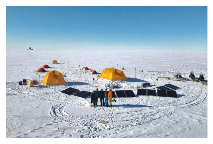
The AES PROFESSIONAL batteries are the energy storage component of the team's (renewable) power system. The system is comprised of solar panels and wind turbines that produce up to 6 kW of solar and 1.6 kW of wind power, which is stored in a 30 kWh battery bank.
